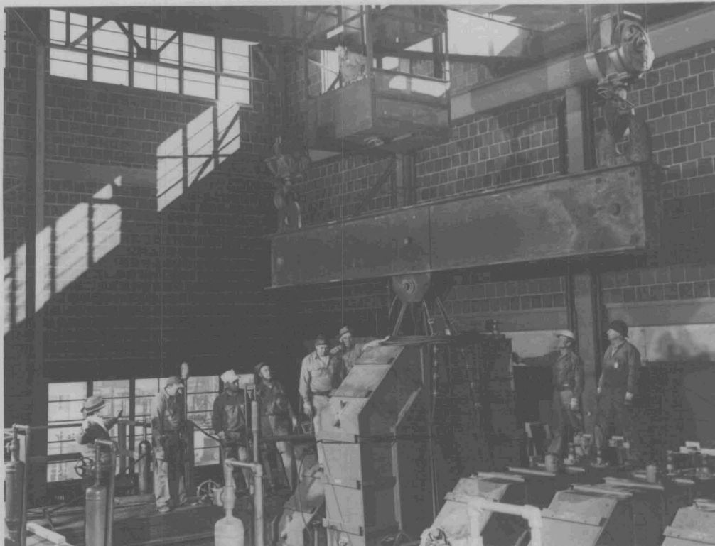
FIGURE 8. TRANSFERRING BETA COIL
