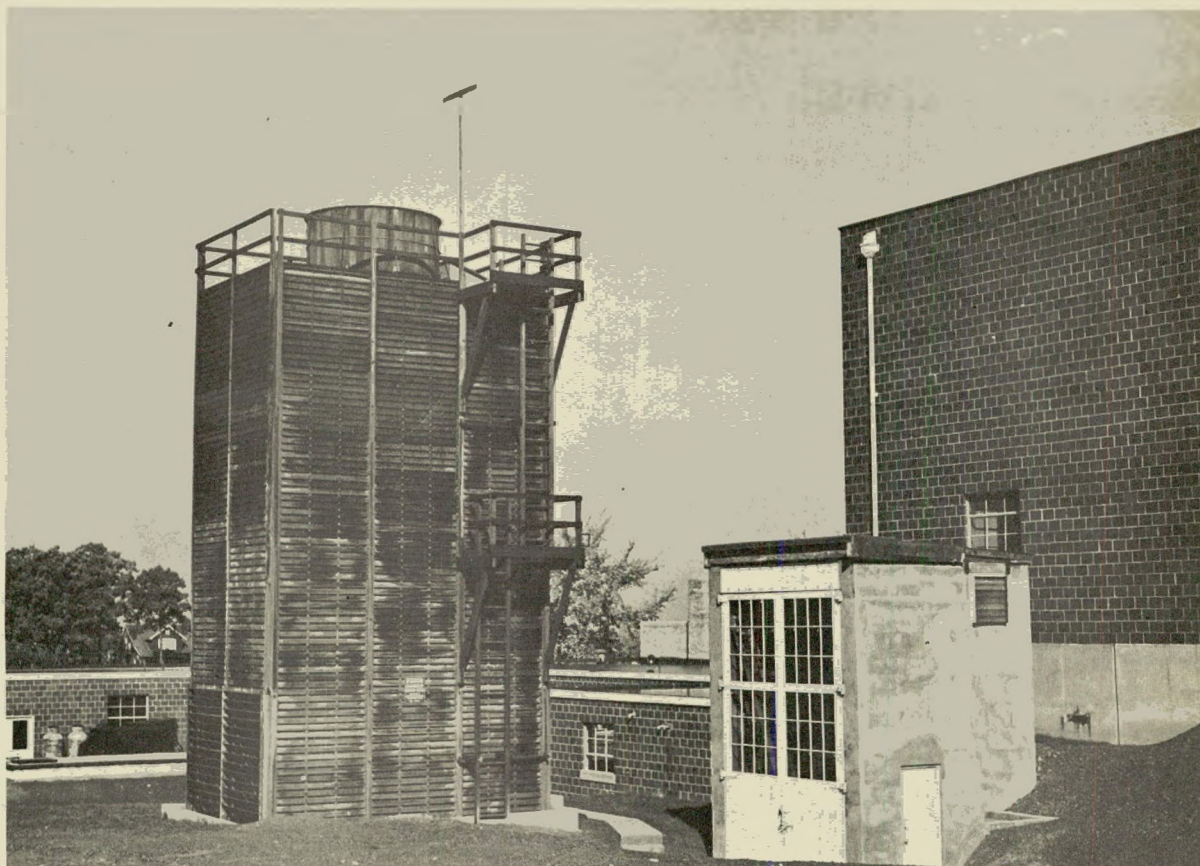
Fig. 16--The cooling tower. The small concrete building at the right houses the homo-polar generator.
