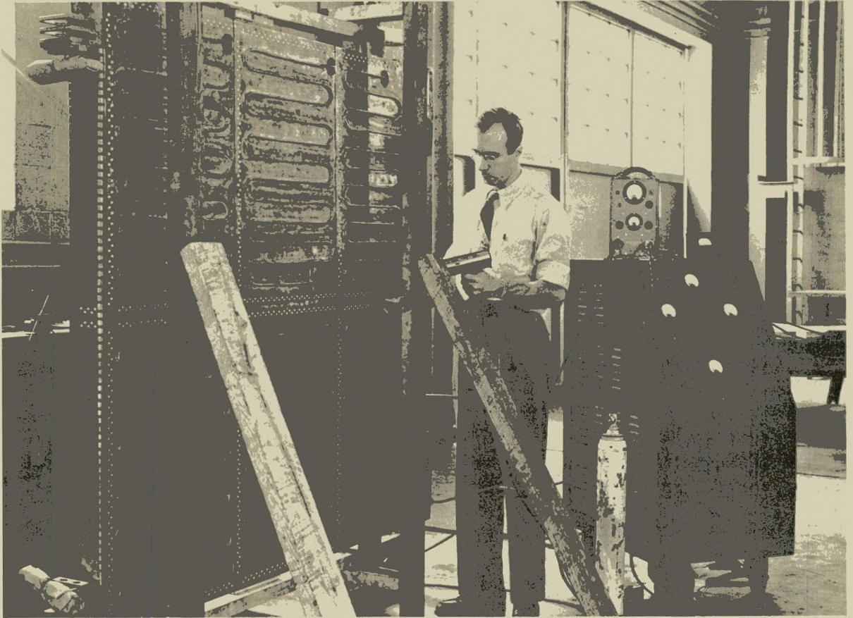
Fig. 4a--Mr. Kearns leak testing the water cooling tubes on the tuning line inner conductor.
